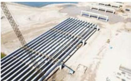
The precaster, who was brought onto the project early due to the use of a Construction Management at Risk contracting method, supplied 204 Type VI-modified AASHTO girders in 17 spans, each approximately 122 ft long, to create the 2067-ft-long bridge.
