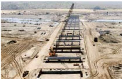
The substructure consisted of cast-in-place drilled shafts, piers, and bent caps.
