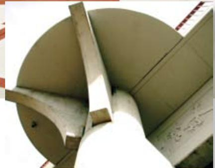
Alcoves with benches were created along the bridge's length to invite pedestrians to linger and enjoy the scenery, while two bat lodgings were created beneath the bridge to accommodate up to 8000 bats. The alcoves along the bridge are each supported by two precast concrete corbels, which served as falsework during construction, reducing project cost and construction time.
