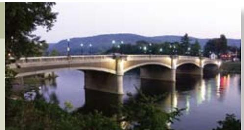
The Hickory Street Bridge in Warren, Pa., replaced an older concrete spandrel arch bridge with four prestressed box-girder spans that replicated the original look and included period lighting, architectural railings, and façade panels.
