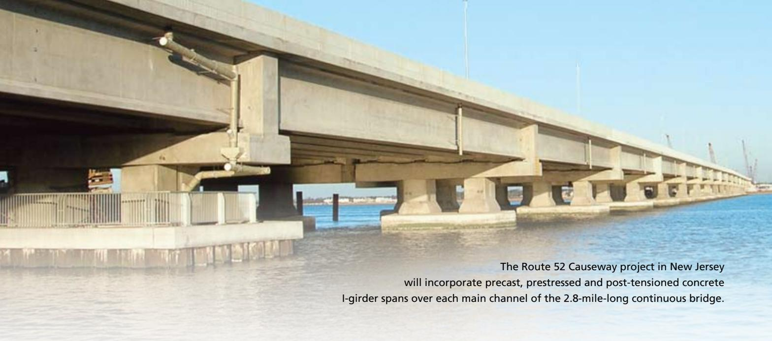
The Route 52 Causeway project in New Jersey will incorporate precast, prestressed and post-tensioned concrete I-girder spans over each main channel of the 2.8-mile-long continuous bridge.
